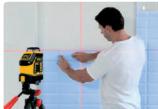
CERAMIC TILE INSTALLATION
