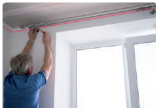
CURTAINS ROD INSTALLATION
